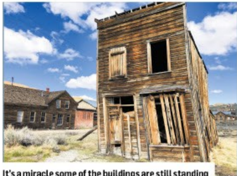
It's a miracle some of the buildings are still standing
